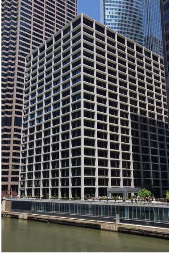
Hartford Building at 100 S. Wacker Dr. (1961; Skidmore, Owings & Merrill)
